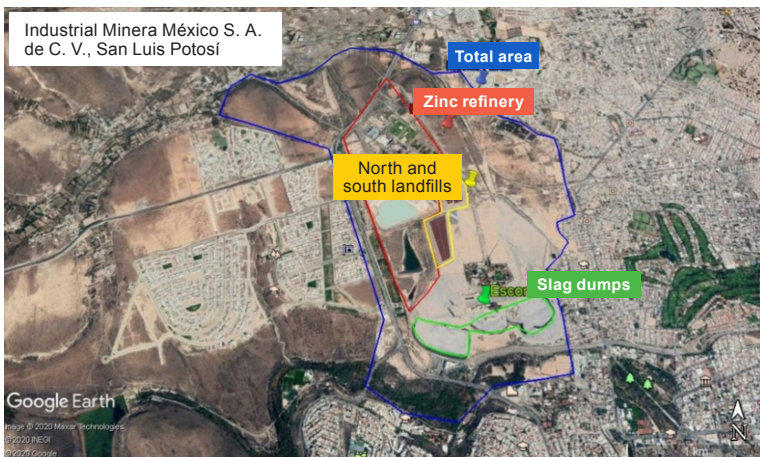
Image VI.7 Metallurgical complex of Industrial Minera México S.A. de C.V. in San Luis Potosí
