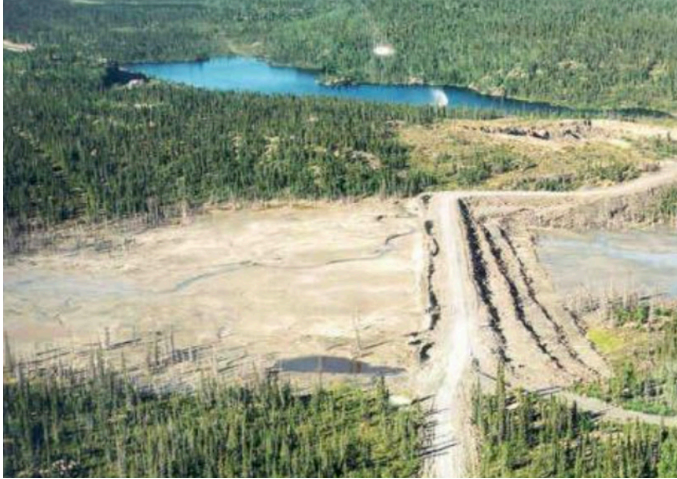
Image VI.3 Tailings dam with dike
