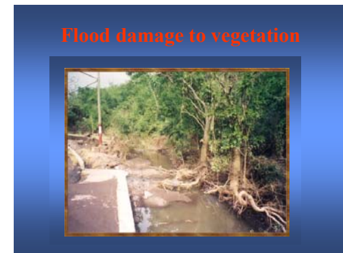
Photo 19: Flood damage to vegetation
