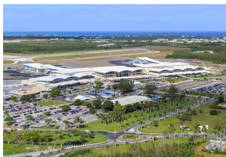
Lynden Pindling International Airport in Nassau, Bahamas.
