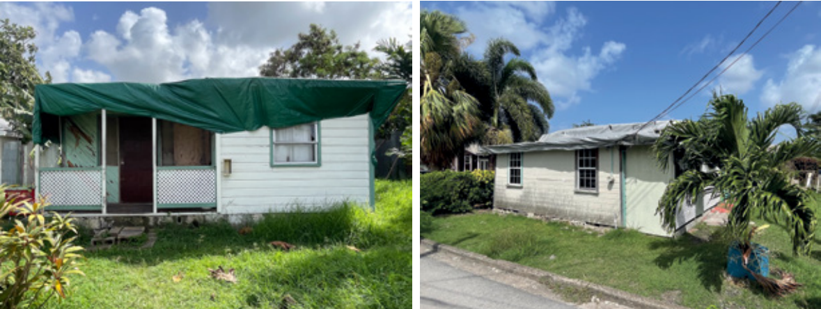
Image 1 Damaged houses with roofs blown off
