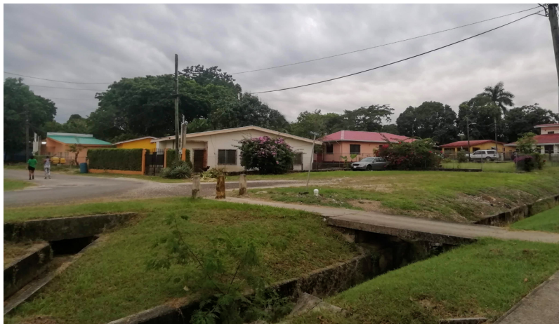
Image 3 Stormwater drainage system plays a critical role in flood prevention
