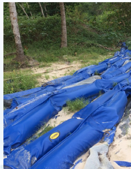
Figure 6: Retention Boom for Controlling Beaching of Sargassum, Saint Lucia, 2018
