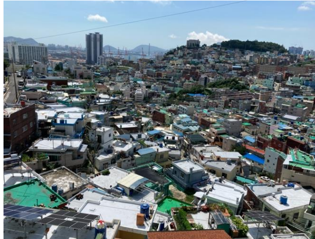
Image 5 Cool roof: Hocheon village (B)
