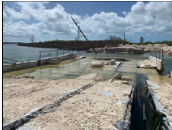
FIGURE 48. COLLAPSED BRIDGE IN NORTH ABACO
