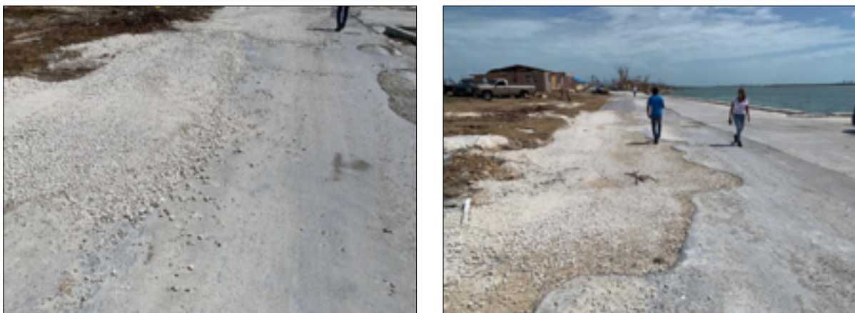
FIGURE 46. DAMAGED ROAD ON GRAND BAHAMAS ISLAND
