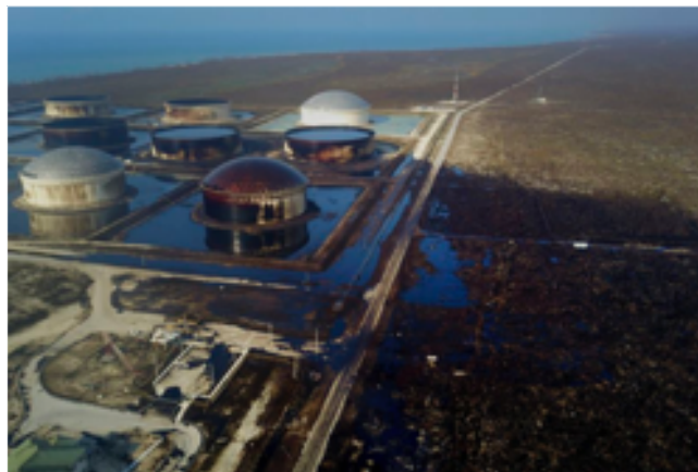
FIGURE 61. SPILL AT SOUTH RIDING POINT OIL STORAGE FACILITY GRAND BAHAMA
