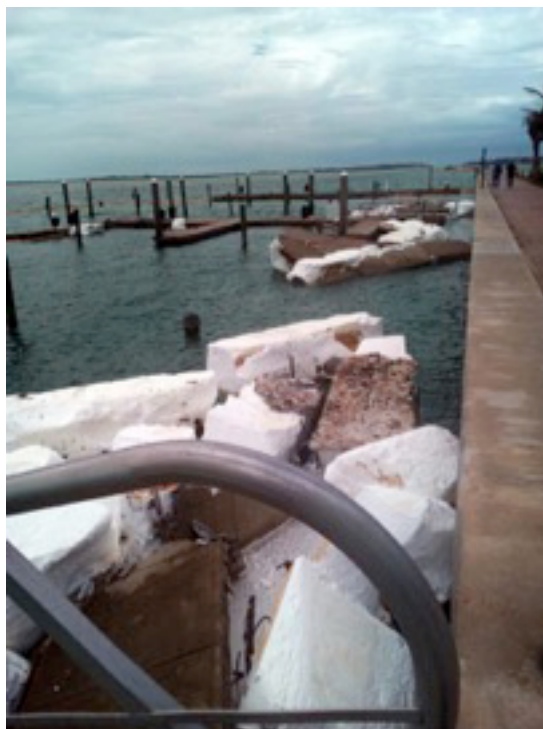
Image 17- Damage to floating docks
