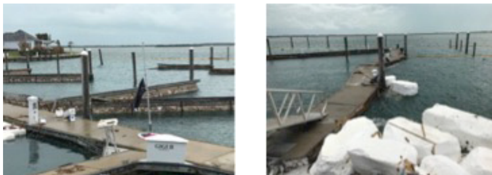
Image 5 - Damage at Resort World Private Marina (Bimini)
