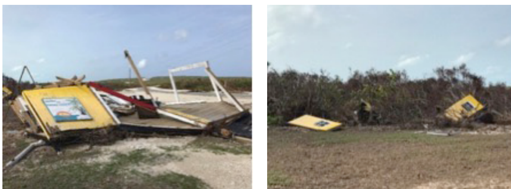
Image 11 - Collapse of Ragged Island airport terminal
