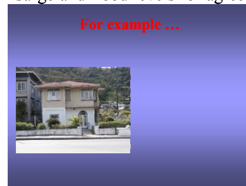
Photo 9: House vulnerable to hurricanes
