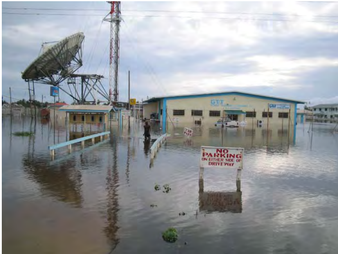
Photo 9 Damage to telecommunications building
