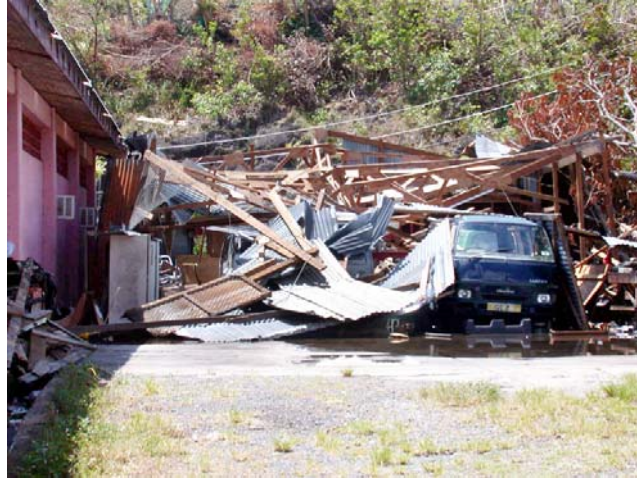
Damage to housing infrastructure, Hurricane Ivan, Grenada: September 2004
