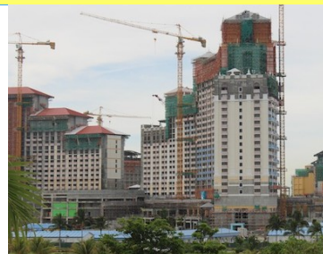
Hotel construction in the Caribbean.
