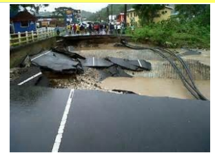
A collapsed road in Saint Lucia in December 2013.
