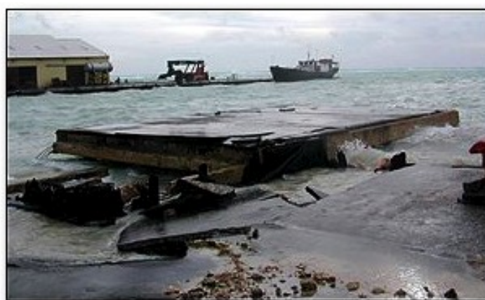
Remnants of a pier damaged by 1999's Hurricane Lenny. Image : BBC World News Online.
