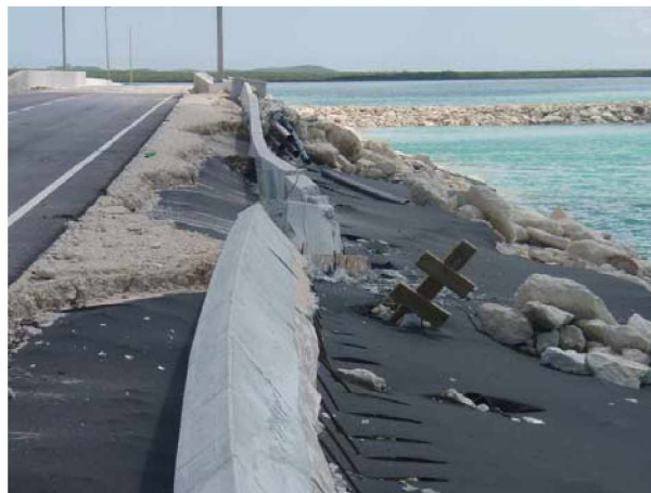
Damaged Causeway – Exposed Geo-textile Fabric
