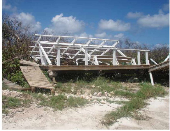
Damaged Boat Landing
