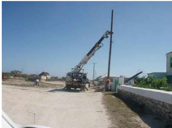
TCU crews at work replacing poles
