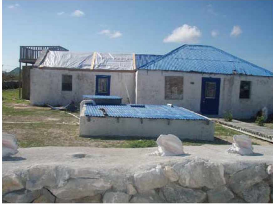
Damage to roof of house on Salt Cay
