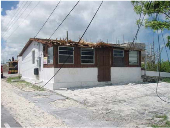
Typical roof damage in North Caicos
