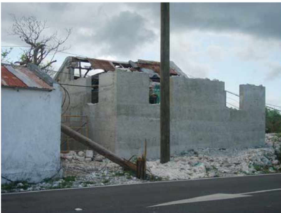
Typical roof damage in North Caicos
