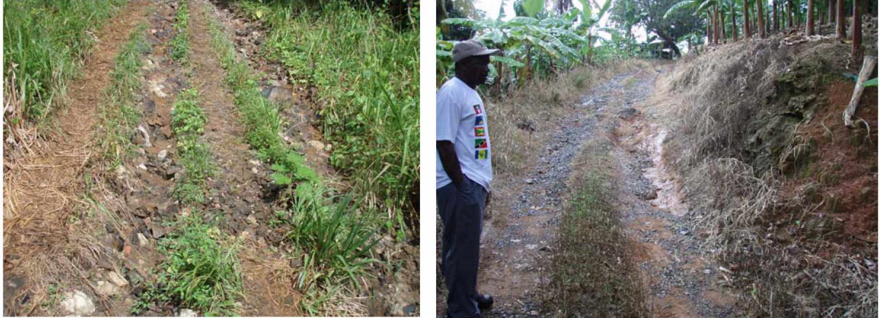
Typical condition of feeder roads after Hurricane Dean
