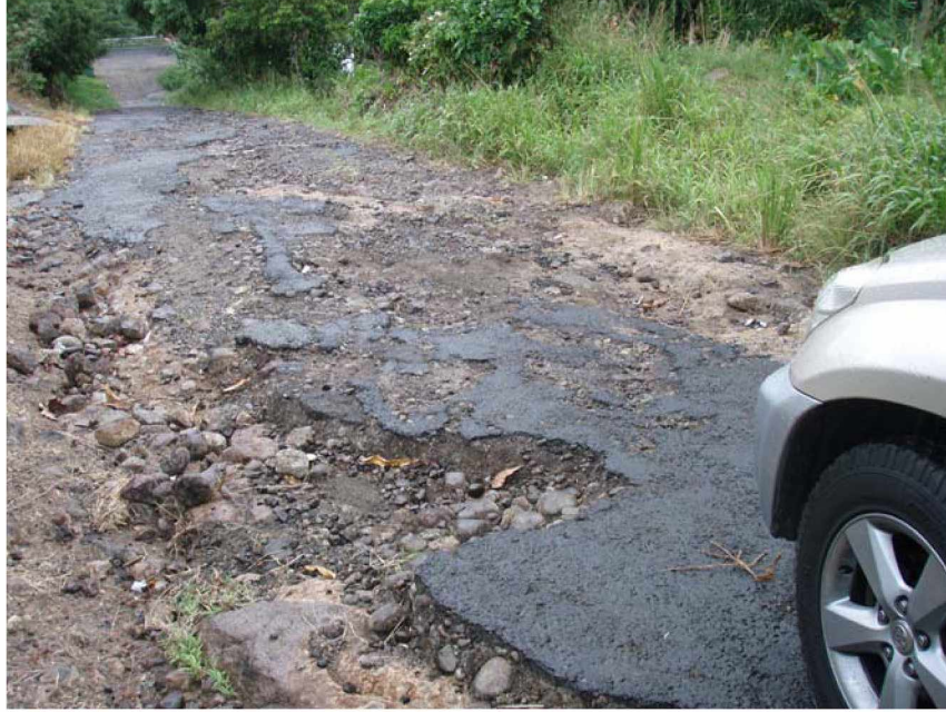
Breakdown of pavement on feeder road after Hurricane Dean
