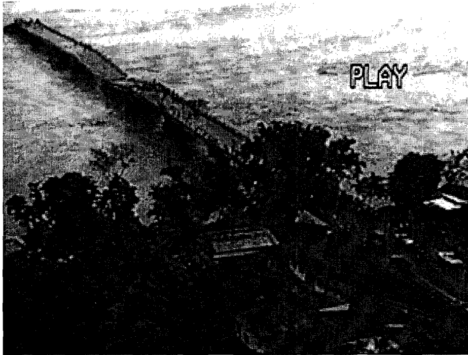
Photo 4. Destroyed bridge in the department of Colón.
