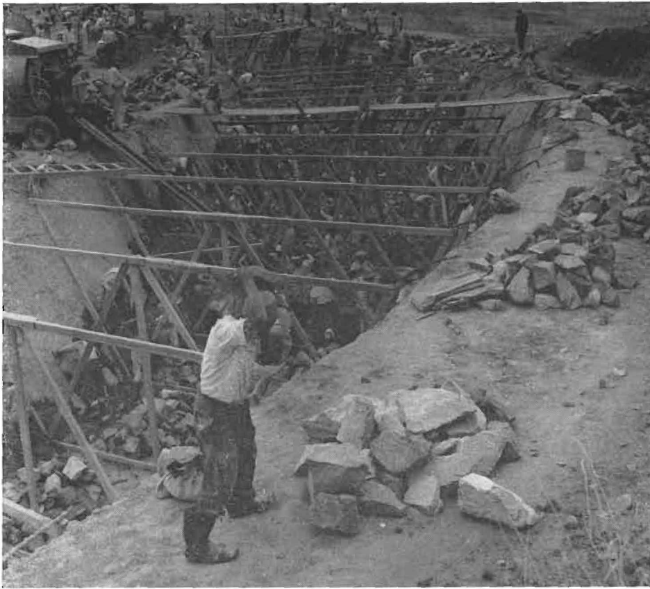
Constructing an irrigation canal in Peru
