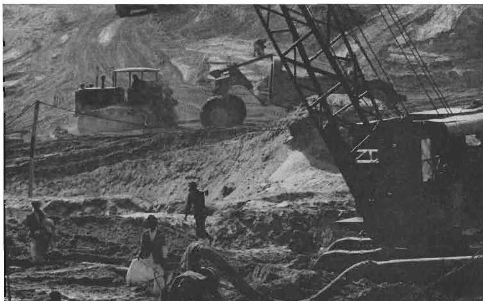
A major irrigation work in Pakistan: Clearing the ground at the Gudu barrage construction site on the Indus River
