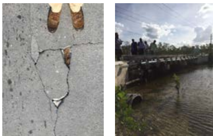
Figure 9- Affected bridge, Conch Sound vicinity
