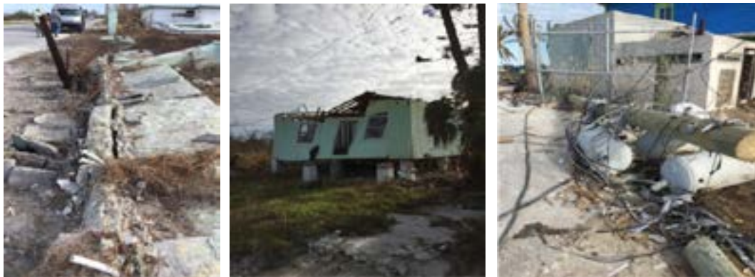
Figure 4- Photos showing front walls, buildings and other major damage caused by storm winds and surge flooding in West End
