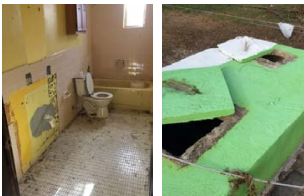
Figure 12- Bathroom and septic tank system affected by flooding in the West End settlement
