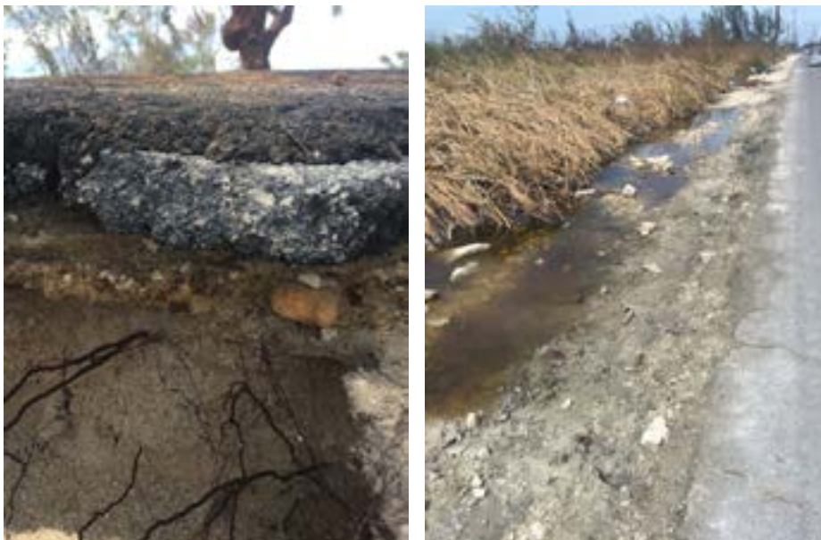
Figure 6- Pavement structure and draining problems, South Beach San Andreas
