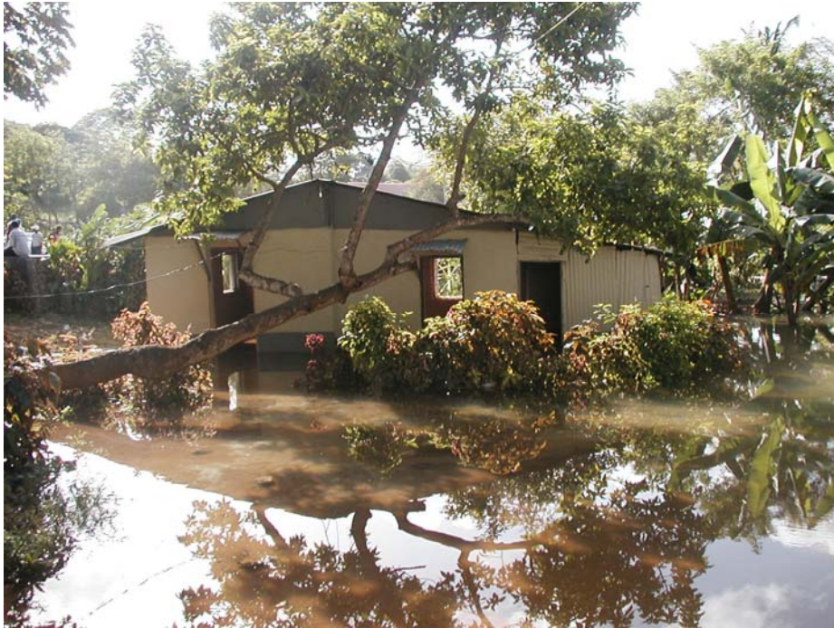
Photo # 7: Evidence of water table that rose above grade at Content, Manchester. Several Houses including this one were flooded.
