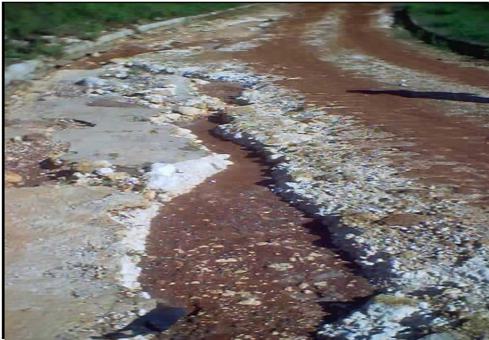
Erosion of roadway
