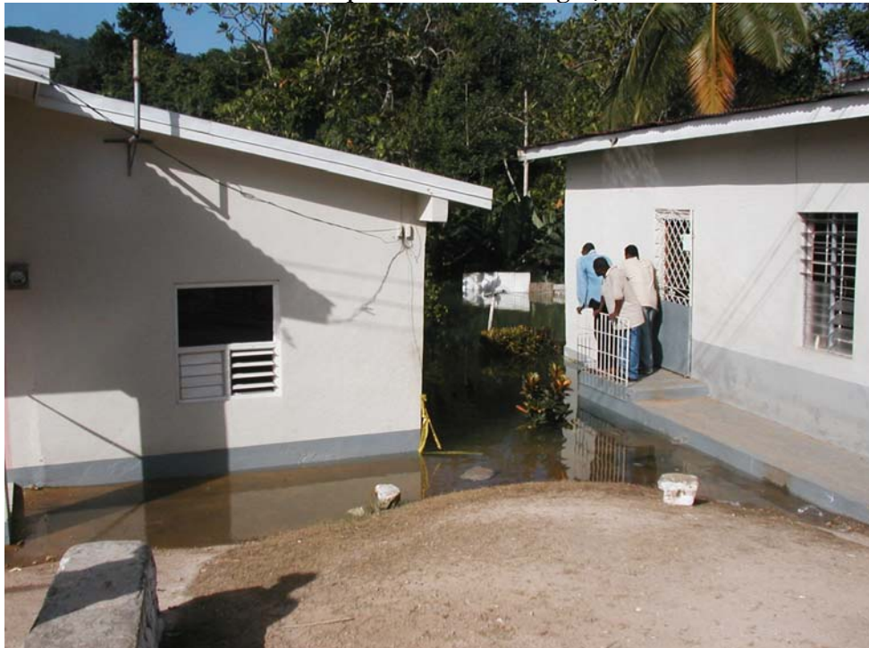
Photo #10: House with inadequate floor level height, Manchester
