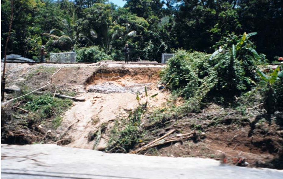
Photo #1: Eroded bank of railway line by the Milk River
