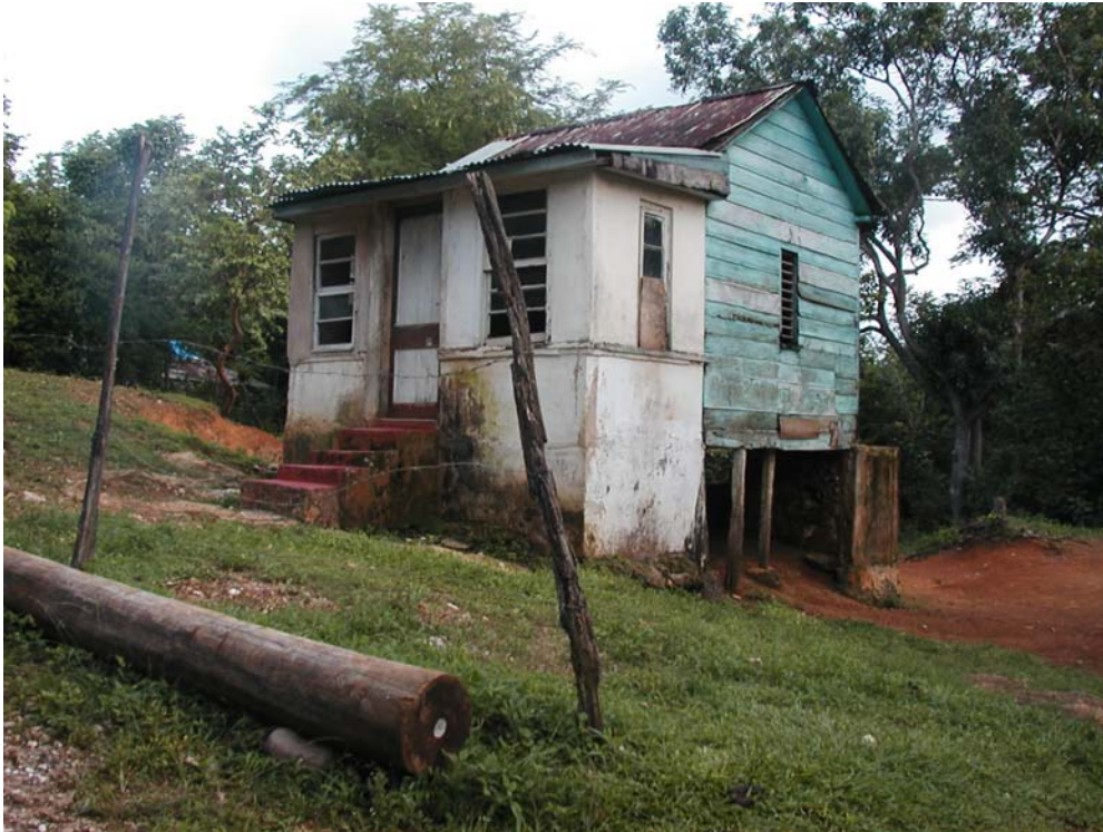
Photo #9: Older house with adequate floor level elevation, Clarendon
