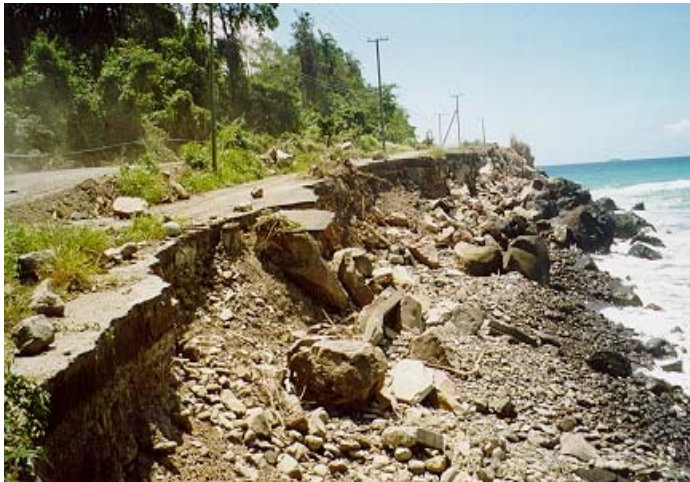
Photo 15: Main road on west coast of Grenada following Hurricane Lenny
