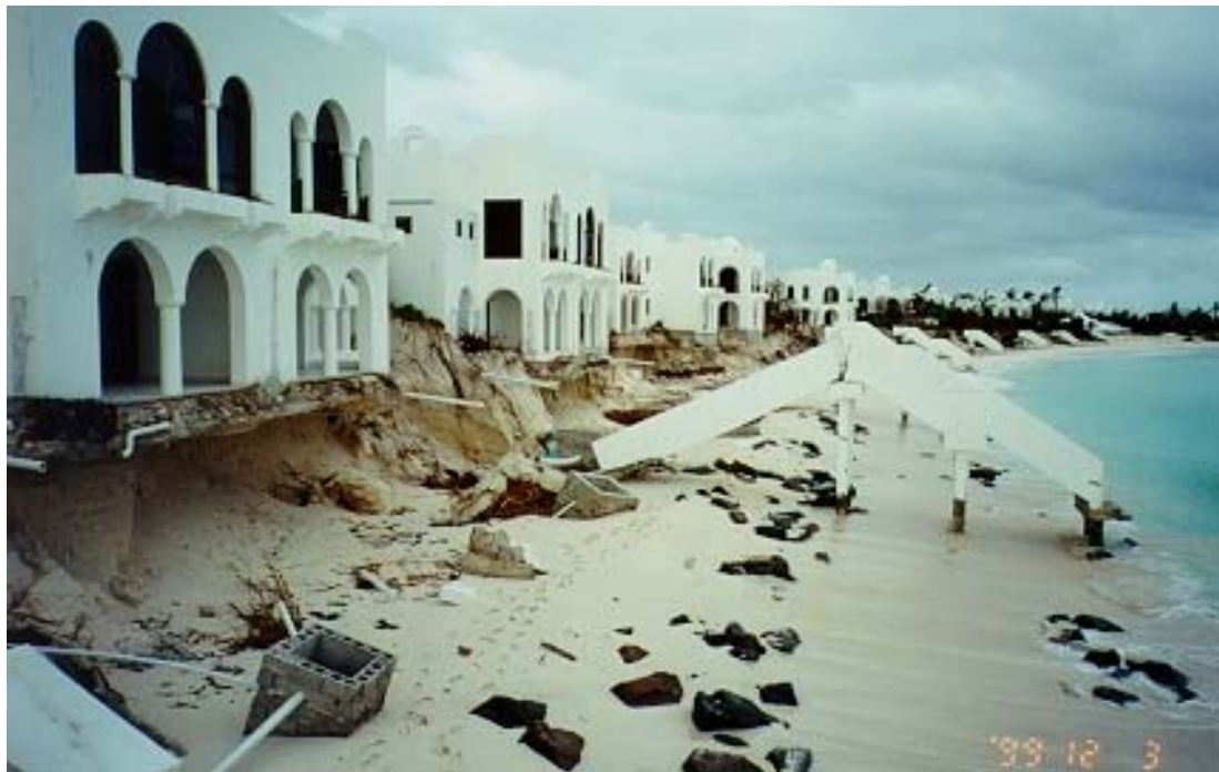
Photo 17: Severe erosion at hotel in Anguilla following Hurricane Lenny
