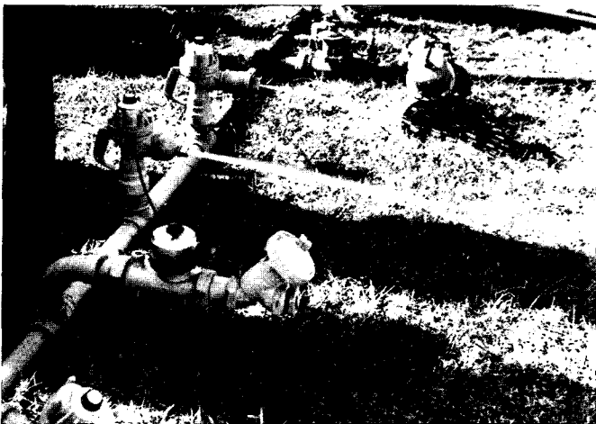
Fig. 5. Automatic water meters for quantity and flow control.
