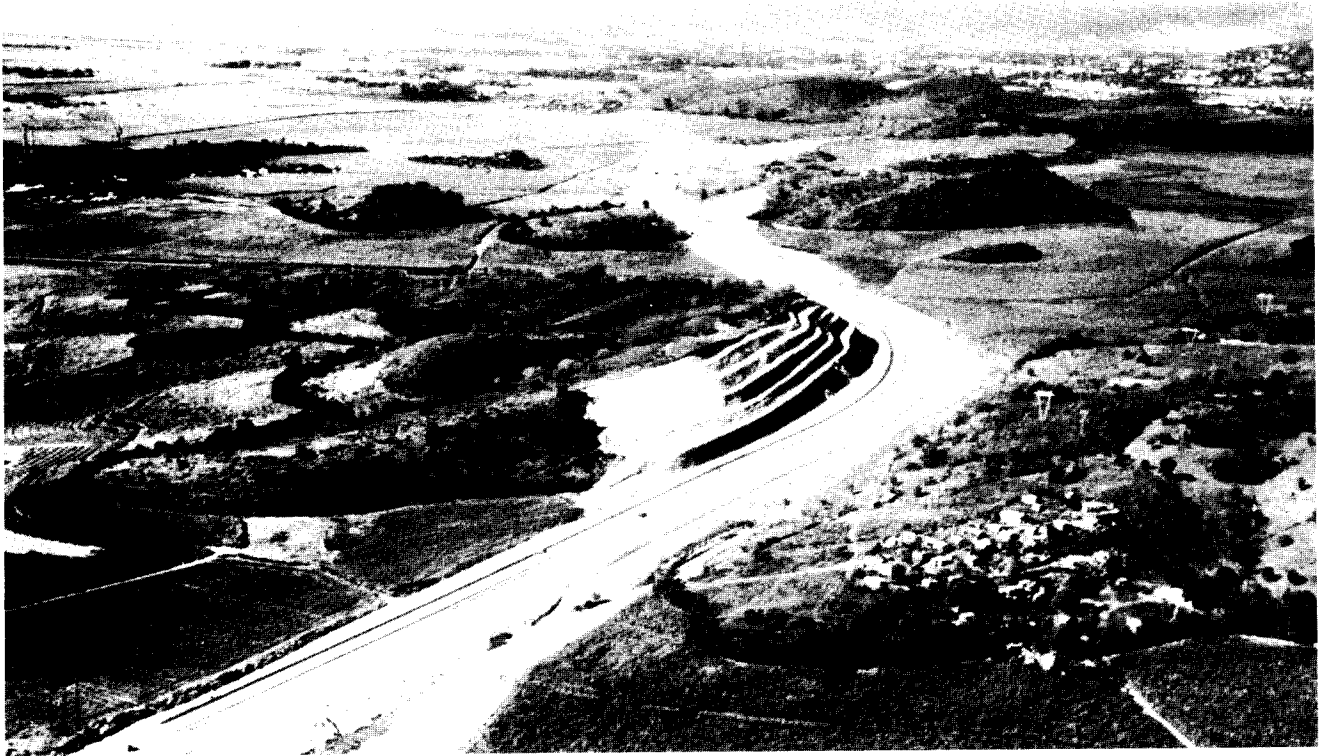
Highway networks are needed to connect the growing urban areas in the islands. Roadways are cut through the hills, embankments are built; where improperly designed, nature erodes them.
