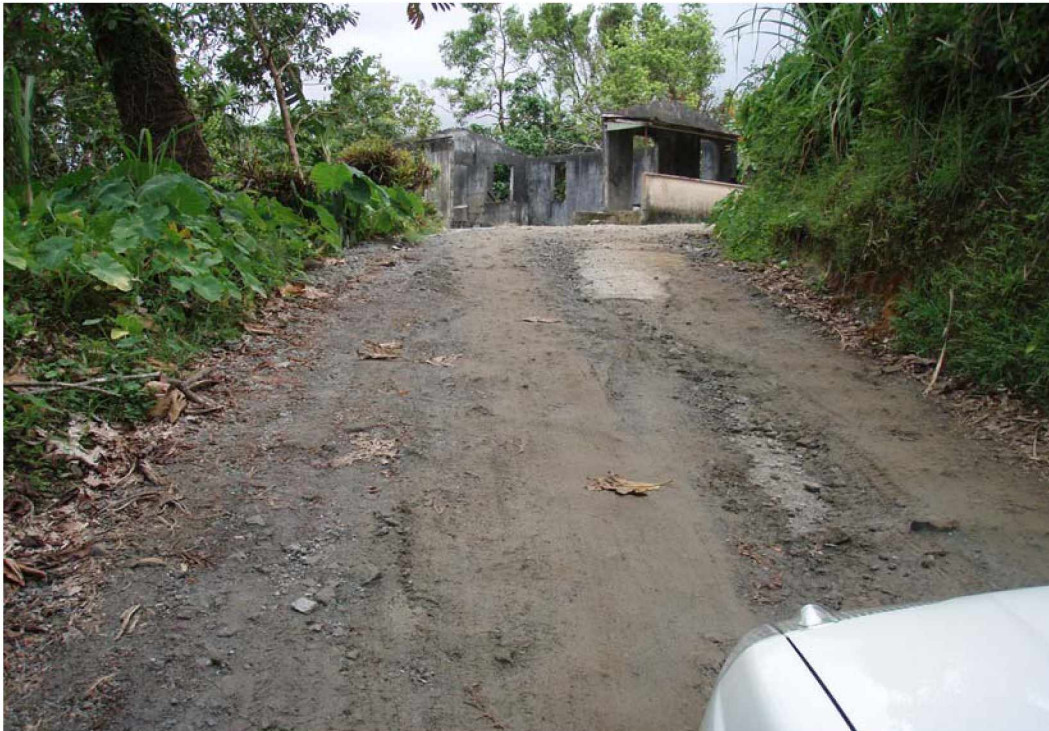
Breakdown of pavement on feeder road after Hurricane Dean
