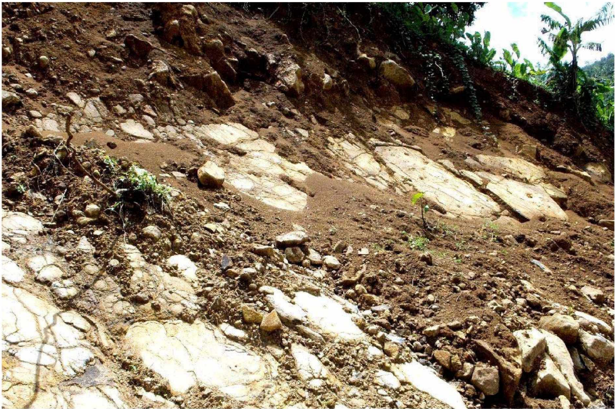
Campbell landslide: Basement Rock cleavage planes parallel to topographic slope at slip surface and perched water table basement strata (Top: left hand side top of scarp, Bottom: right hand side top of scarp).
