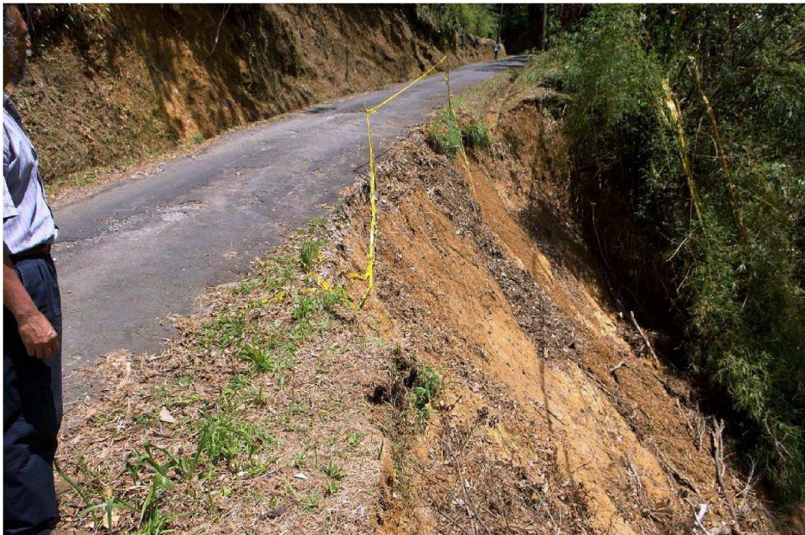
Middleham Falls – Trafalgar Road junction
