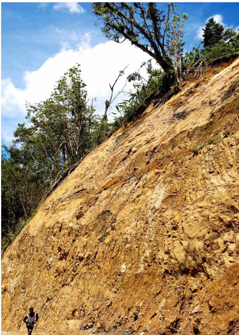
Laudat landslide at highest upslope tree to be removed.
