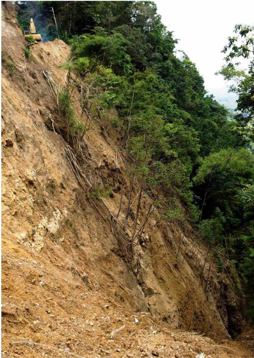
Laudat downslope 60° to bottom of valley 150 m below.
