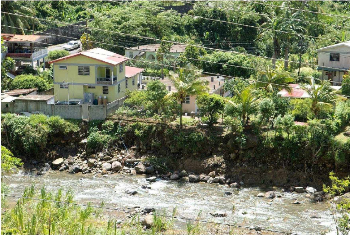
Roseau Valley: River erosion affecting residential communities on south bank.
