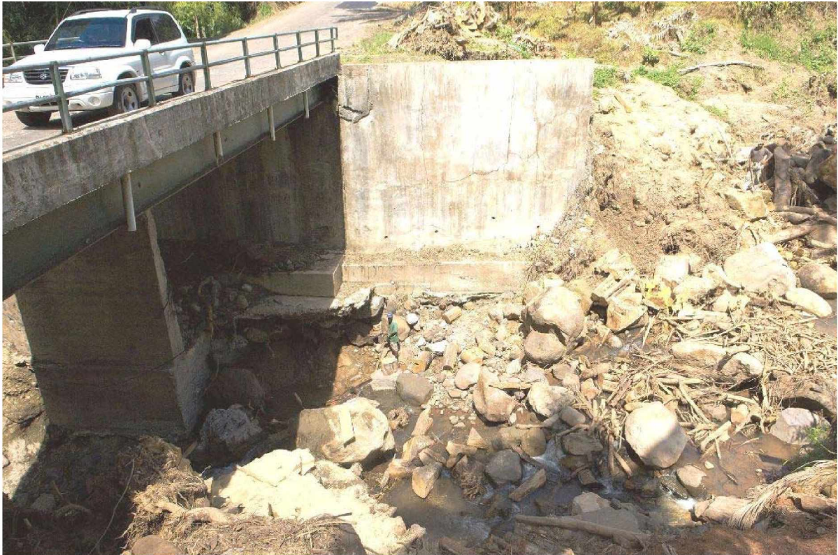
Pont Cassé – Layou Road: Grand Ravine Bridge Foundations undermined.
