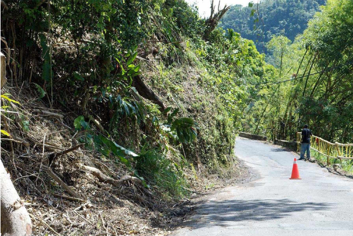
Roseau Valley - Fond Cani: Debris slides up-slope and edge failures and washouts down slope of roadway on blind curve. Slope to be cut and roadway realigned to regain roadway width.
