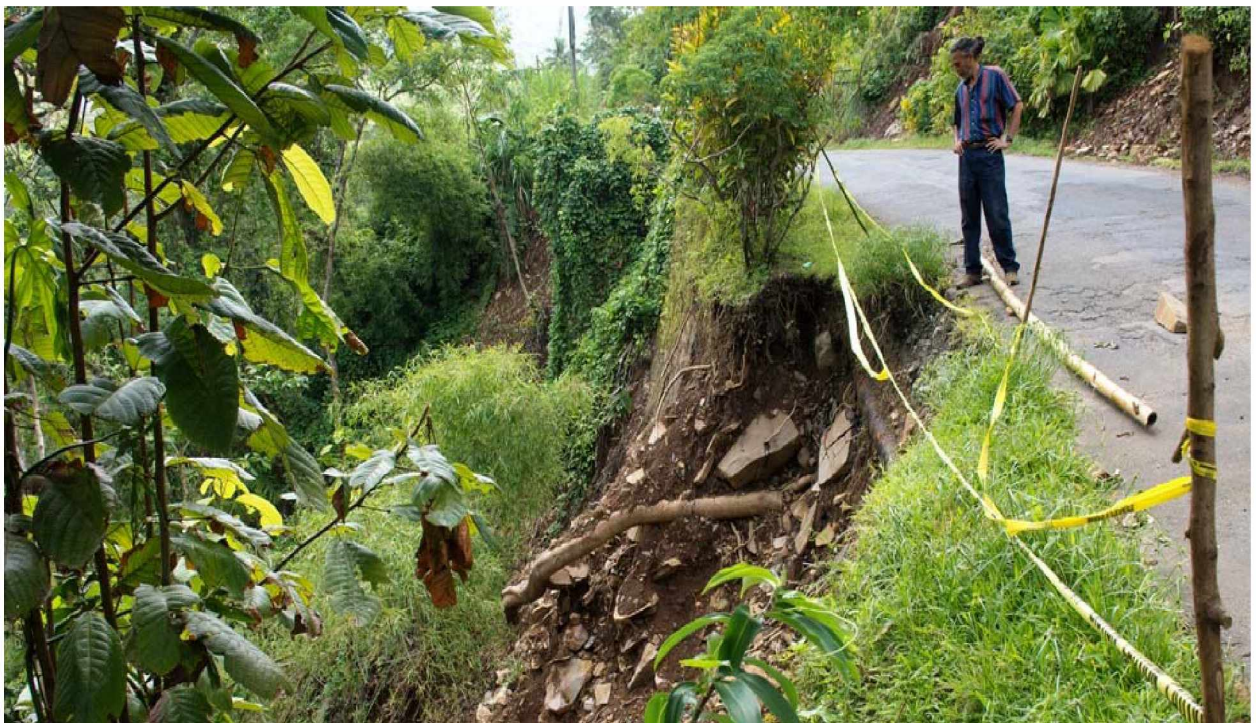
Imperial Road washouts exposing water supply lines
