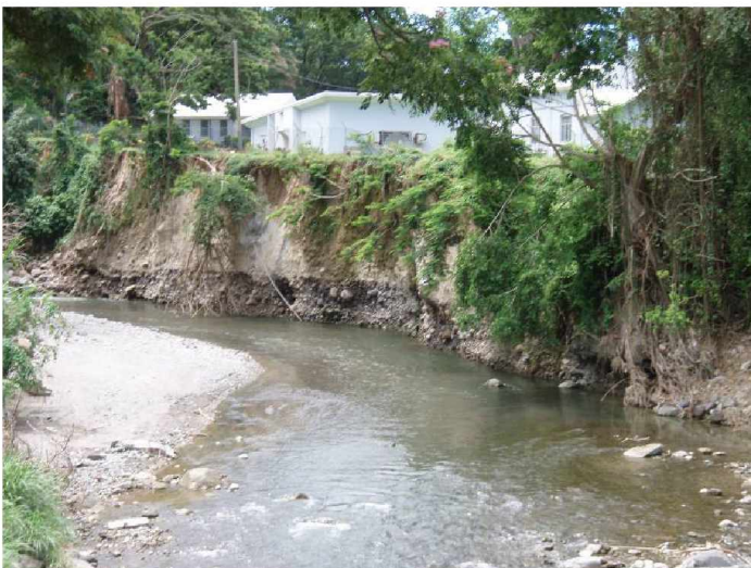
Roseau River induced erosion at UWI Campus
