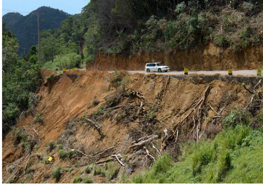
Major landslide on Imperial Highway
